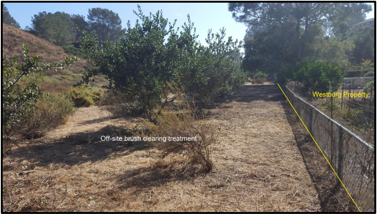
Photo 6. View looking south at off-site Zone 2 fuel modification.
