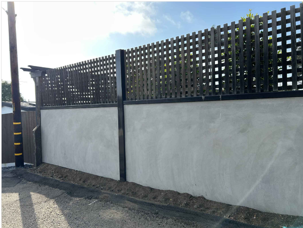
⑯ EXISTING FENCE @ ALLEY
