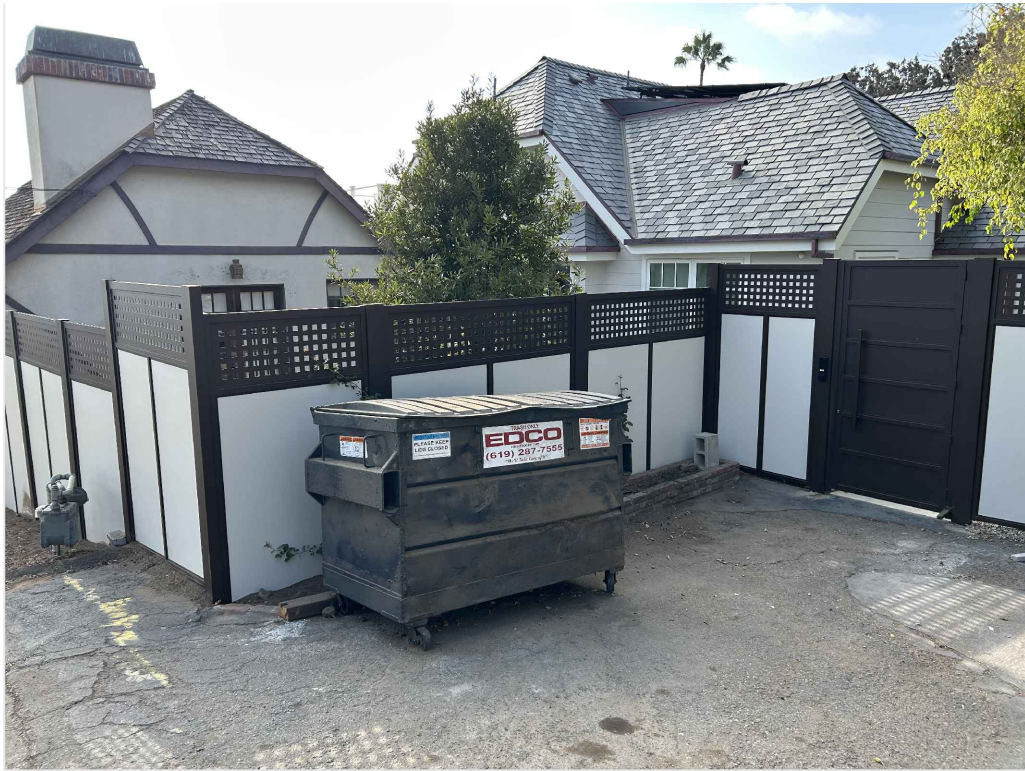
⑪ FENCE AT PARKING STALLS
