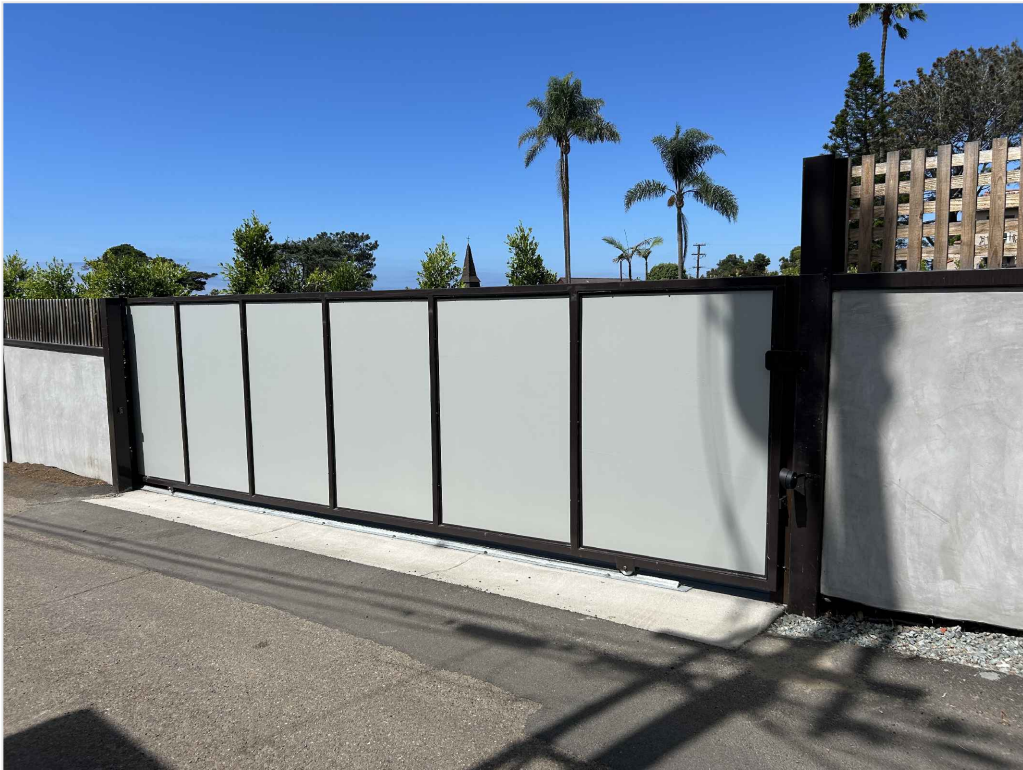
⑭ EXISTING CAR GATE
