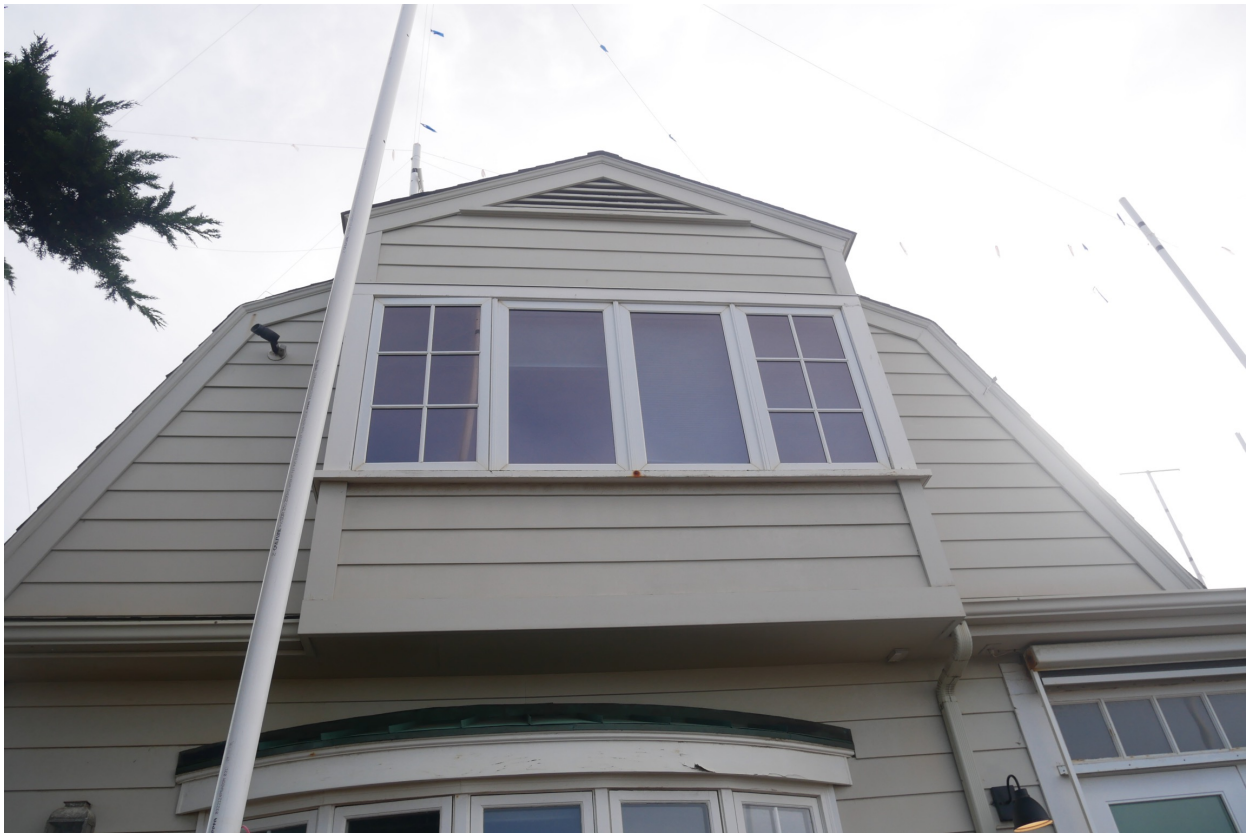
Photograph #12: West Elevation, second floor projection with windows added per City of Del Mar Design Review Board Approval 88-64, 2/22/1995
