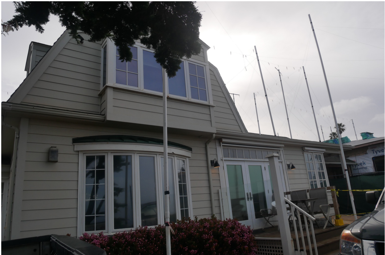
Photograph #11: West Elevation, all windows modified per City of Del Mar Design Review Board Approval 88-64, 2/22/1995
