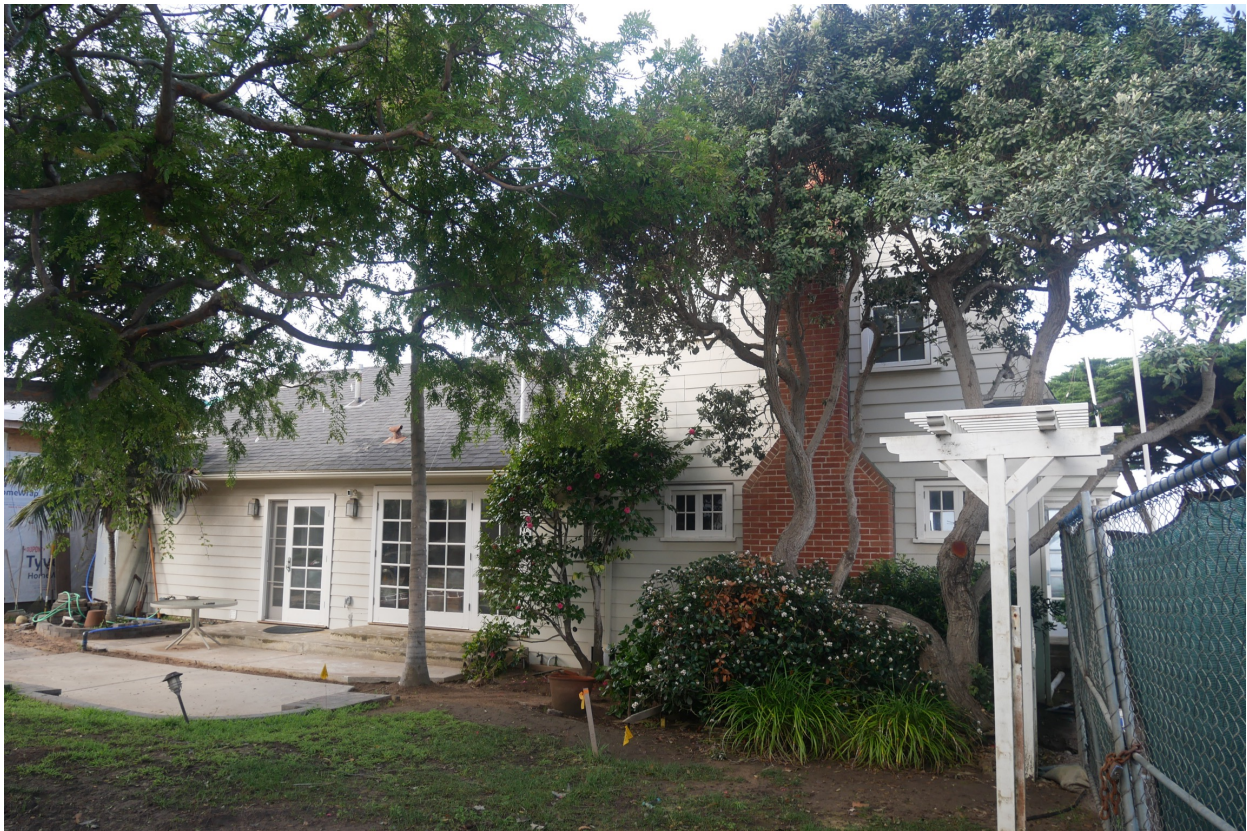
Photograph #16: East Elevation, ground floor porch enclosure with new doors and windows added per City of Del Mar Design Review Board Approval 88-64, 2/22/1995
