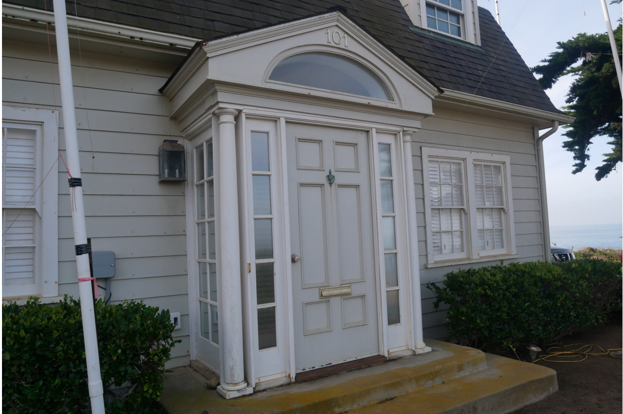
Photograph #8: North Elevation, modified entry vestibule per City of Del Mar Design Review Board Approval 88-64, 2/22/1995
