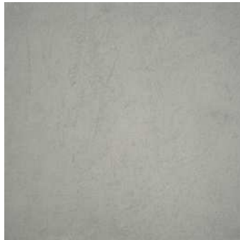
WALLS - Grey Plaster
