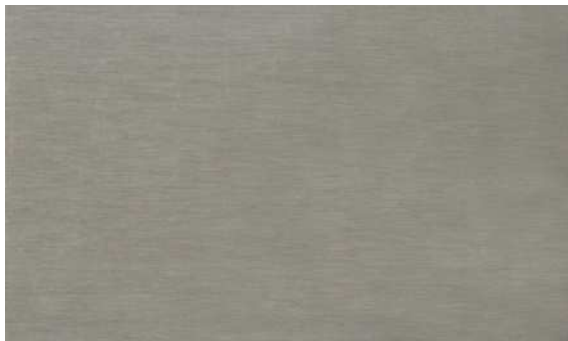
ROOF - VMZ Quartz Zinc
