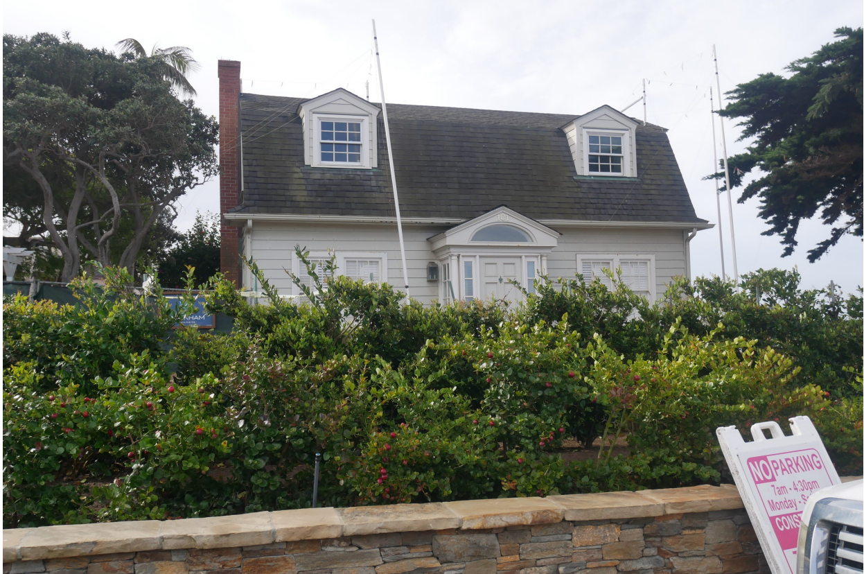
Photograph #6: North Elevation, from 11 th Street
