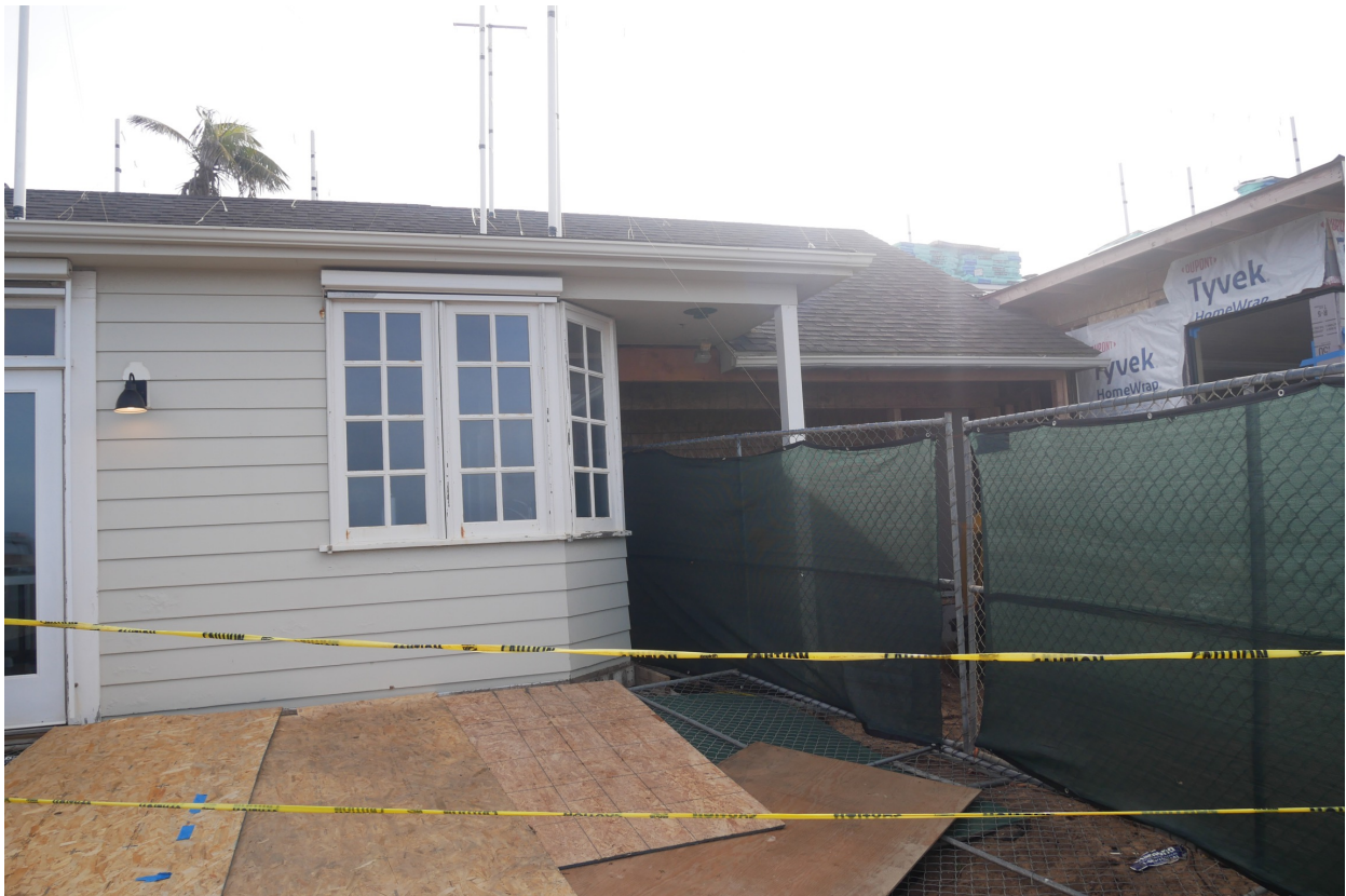
Photograph #15: West Elevation, ground floor porch enclosure added per City of Del Mar Design Review Board Approval 88-64, 2/22/1995 and ADU addition added per City of Del Mar approved building permits 8/15/2023
