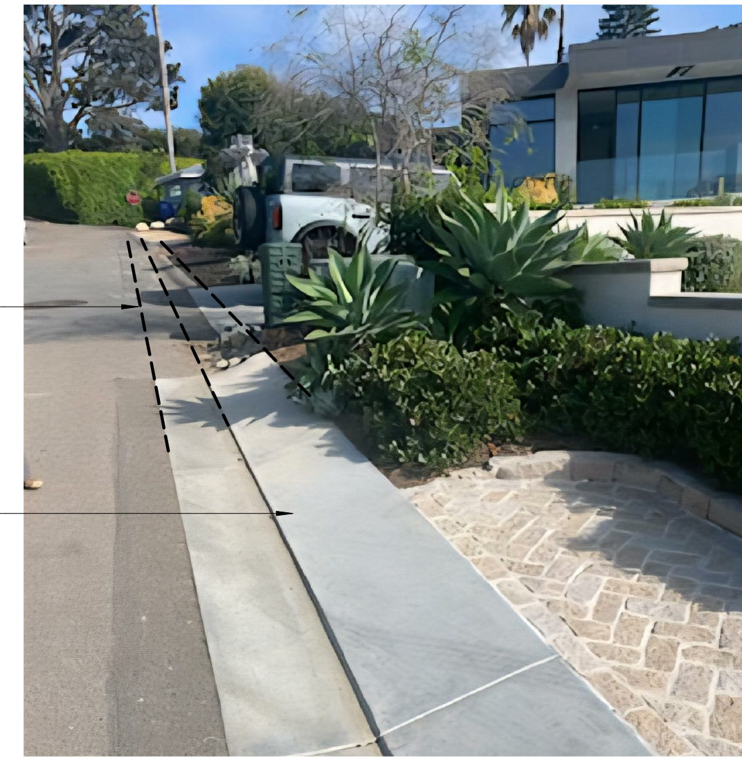
EXISTING CURB AT WEST NEIGHBOR
