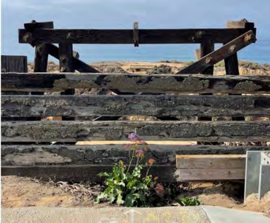
Figure 2 – Remnants of Historic Overcrossing at 10 th Street
