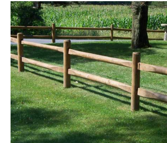
WETLAND BUFFER FENCE
