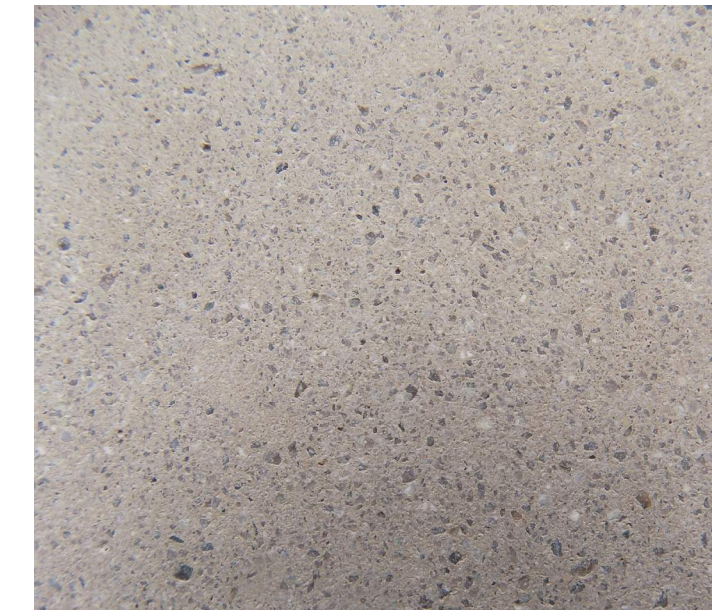
ENHANCED CONCRETE PAVING
