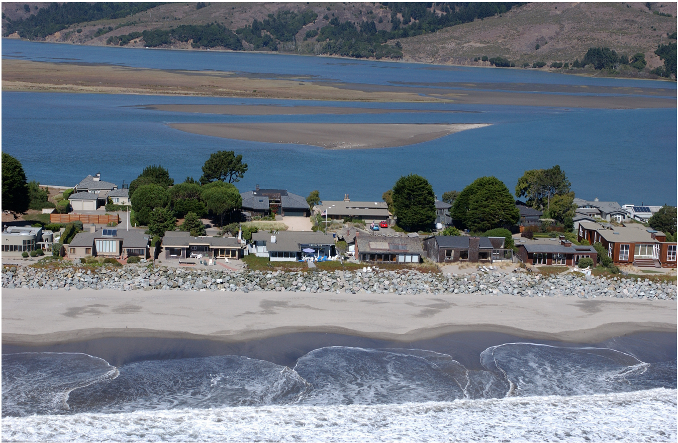
FIGURE 6.7 Developed sand spit at Stinson Beach in Marin County, California, where a revetment has been constructed in an effort to protect the homes. This spit cannot migrate with sea-level rise. SOURCE: Copyright 2002–2012 Kenneth & Gabrielle Adelman, California Coastal Records Project, < www.Californiacoastline.org >.
