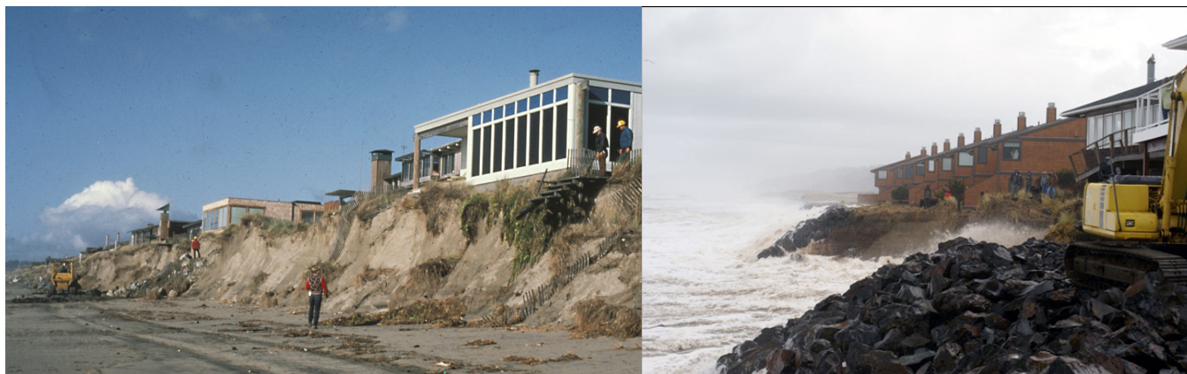
FIGURE 6.9 Construction of private homes on the frontal dunes. (Left) Homes in central Monterey Bay were threatened by erosion during the high tides, elevated sea levels, and large storm wave of the 1983 El Niño. SOURCE: Courtesy of Gary Griggs, University of California, Santa Cruz. (Right) Placement of riprap during storm conditions to protect development on dunes in Neskowin, Oregon. SOURCE: Courtesy of Armand Thibault.
