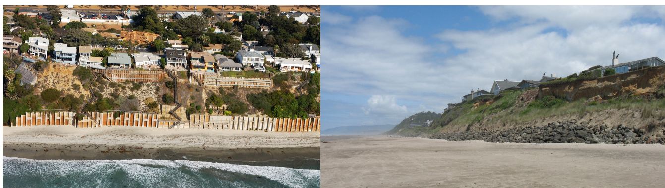
FIGURE 6.4 Seawalls and revetments fronting coastal cliffs and bluffs in California and Oregon. (Left) Concrete and timber seawalls protecting cliff top homes in Solana Beach, California. SOURCE: Copyright 2002–2012 Kenneth & Gabrielle Adelman, California Coastal Records Project, < www.Californiacoastline.org >. (Right) Rip rap protecting bluff top housing along the central Oregon coast. SOURCE: Courtesy of Gary Griggs, University of California, Santa Cruz.
