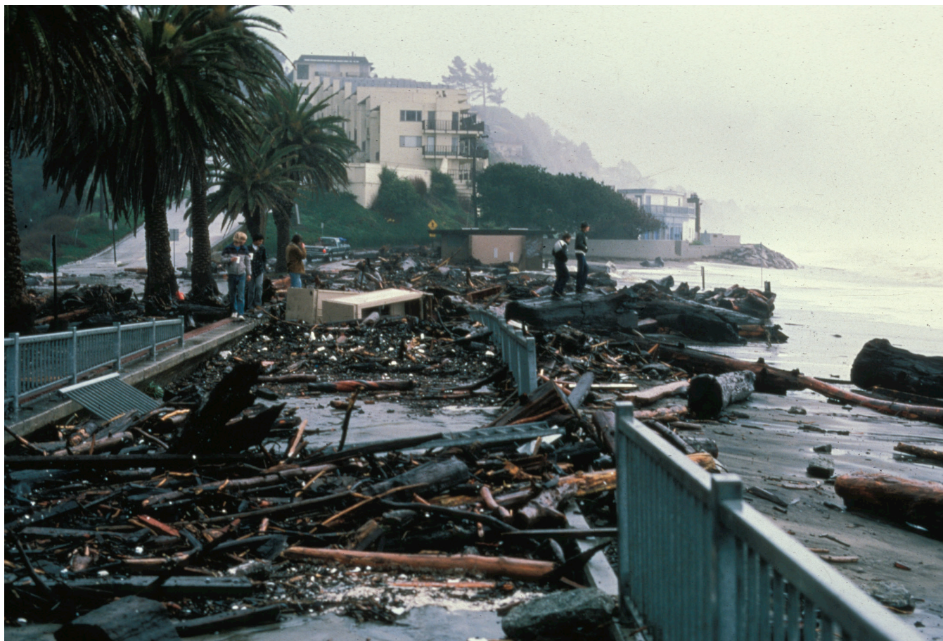
FIGURE 5.11 Rio Del Mar on northern Monterey Bay was damaged during the El Niño winter of 1983 by large waves arriving simultaneously with high tides and elevated sea levels. SOURCE: Courtesy of Gary Griggs, University of California, Santa Cruz.
