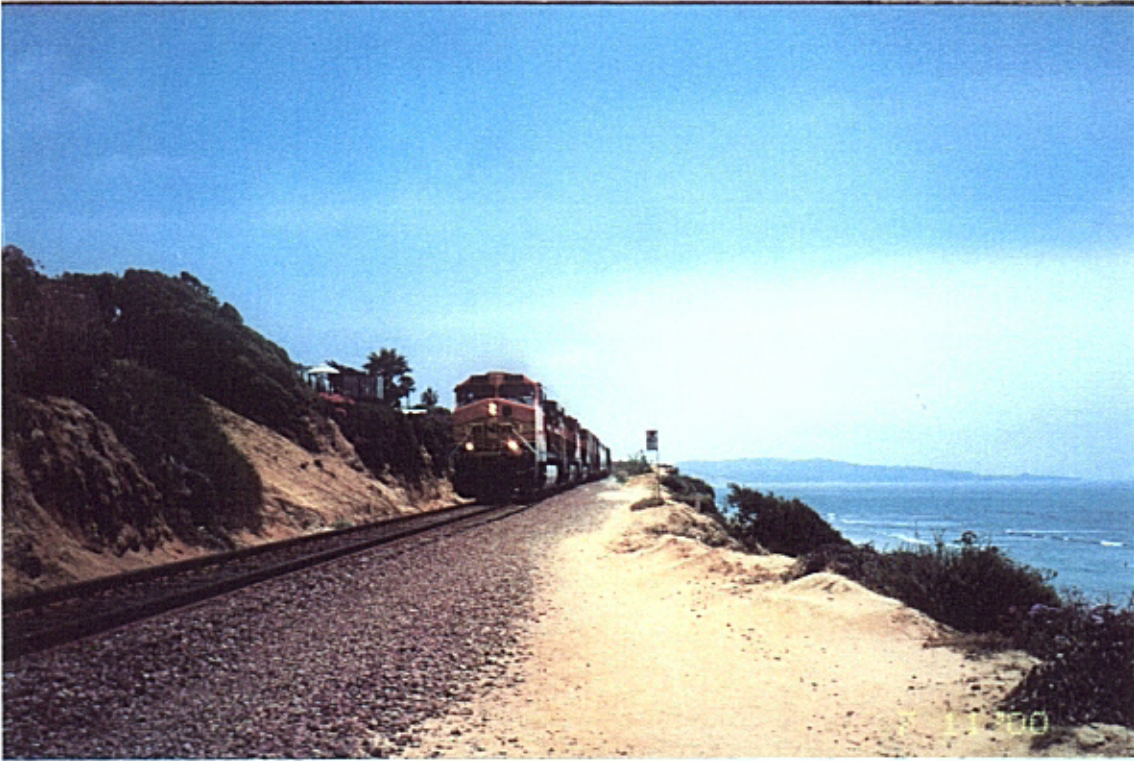
Close proximity of tracks to bluff top, northern section.
