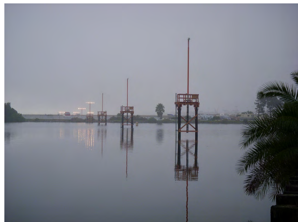
Figure 4.7 West End of Runway (background), San Diego International Airport. 01.19.11, morning : ~7.1 feet above mean low tide.
