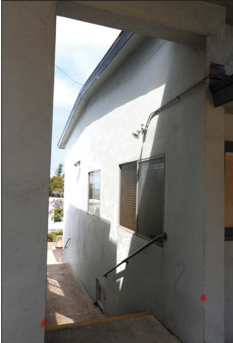
PHOTOGRAPH 13 South Wall of Building B Showing Windows
