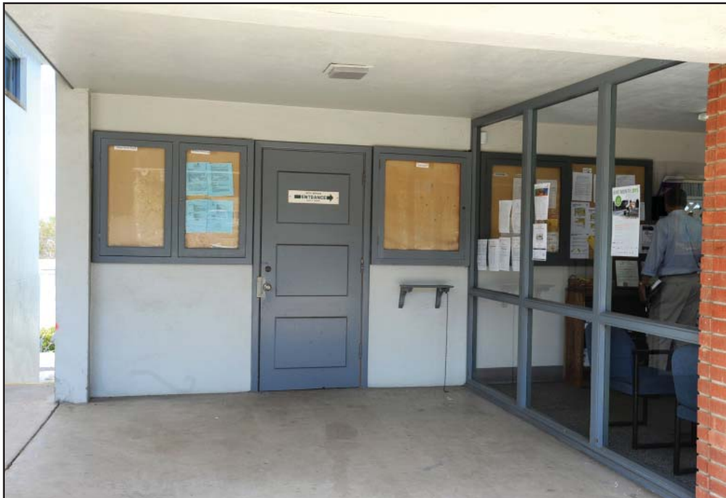
PHOTOGRAPH 12 Building B, South End of Façade
