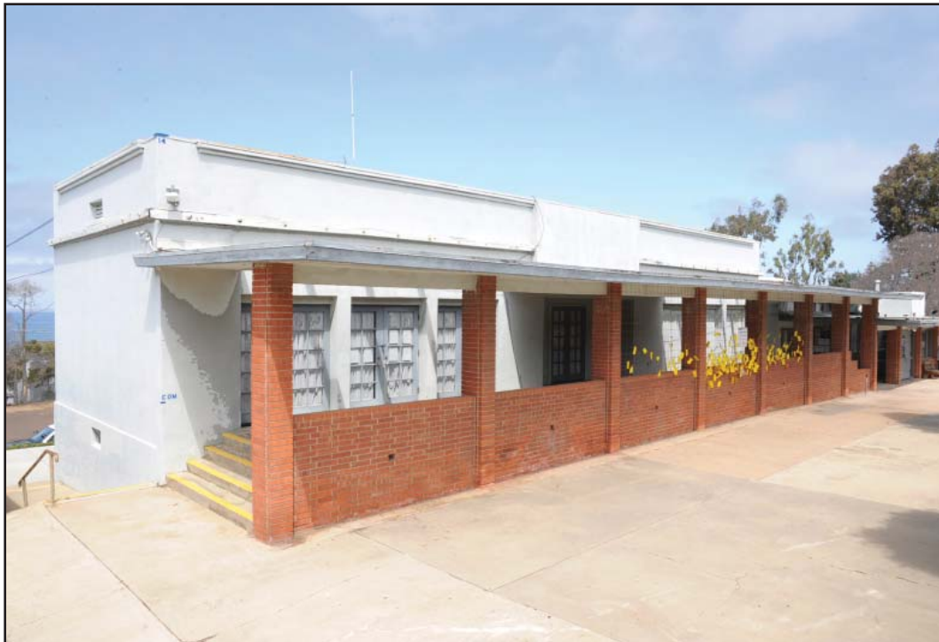
PHOTOGRAPH 2 Building A, Façade Looking Northwest
