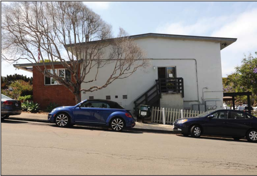
PHOTOGRAPH 14 North Wall of Building B
