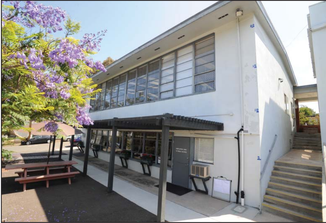
PHOTOGRAPH 16 West Wall of Building B, Looking Northeast
