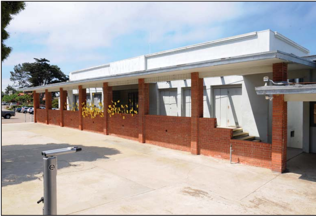
PHOTOGRAPH 1 Building A, Façade Looking Southwest
