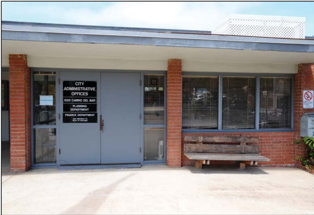
PHOTOGRAPH 11 Front Door of Building B
