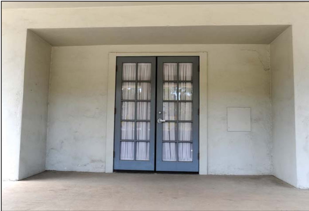
PHOTOGRAPH 3 Building A, Front Door
