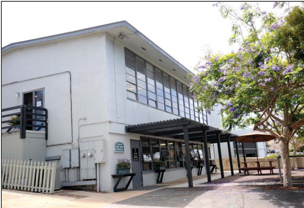
PHOTOGRAPH 15 West Wall of Building B, Looking Southeast
