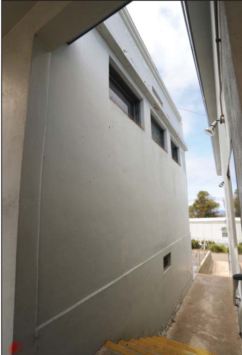
PHOTOGRAPH 6 North Side of Building A
