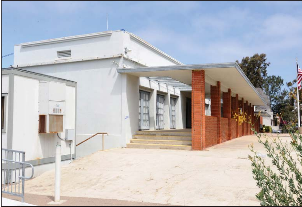
PHOTOGRAPH 5 Building A Portico, Looking Northwest
