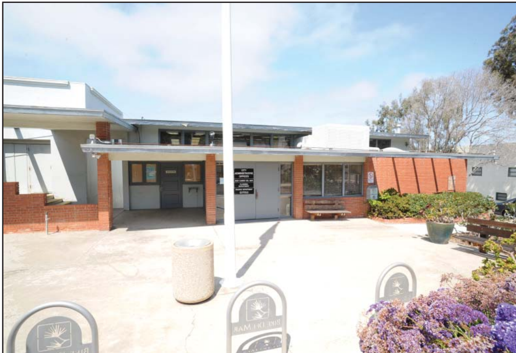
PHOTOGRAPH 10 Building B Façade, Looking West
