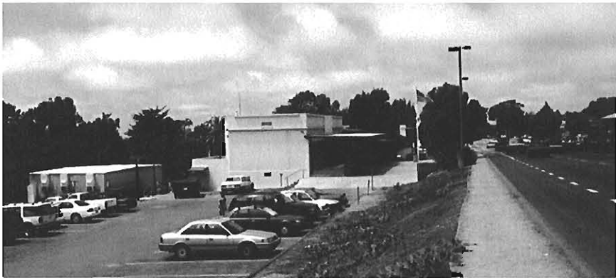
City Hall site envisioned for expansion of city services and public gathering space
