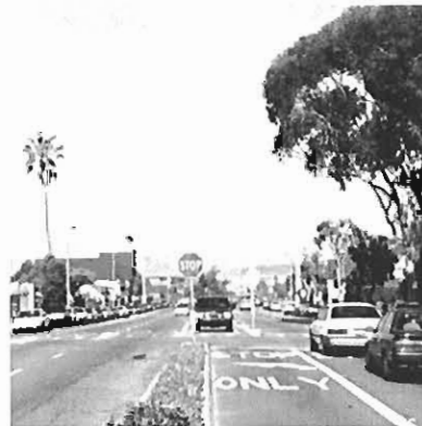
Left turn lane at 13th Street
