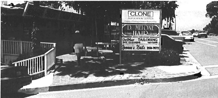
Existing ramp configuration at the northwest corner of 12th Street and Camino del Mar
