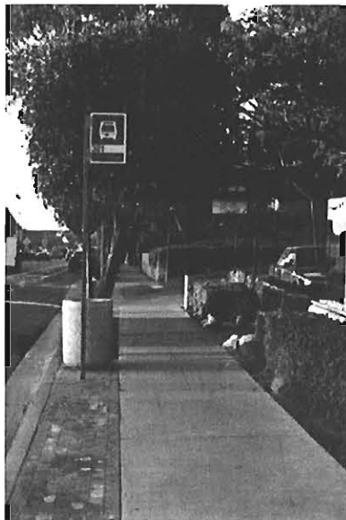
Concrete path of travel with brick
