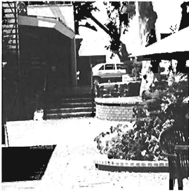
Segments of the path of travel requiring modifications for accessibility
