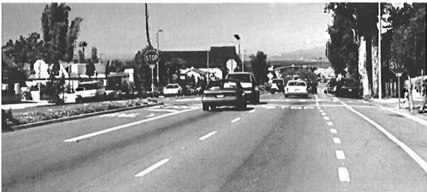
Camino del Mar roadway with automobile, bicycle and parking lanes
