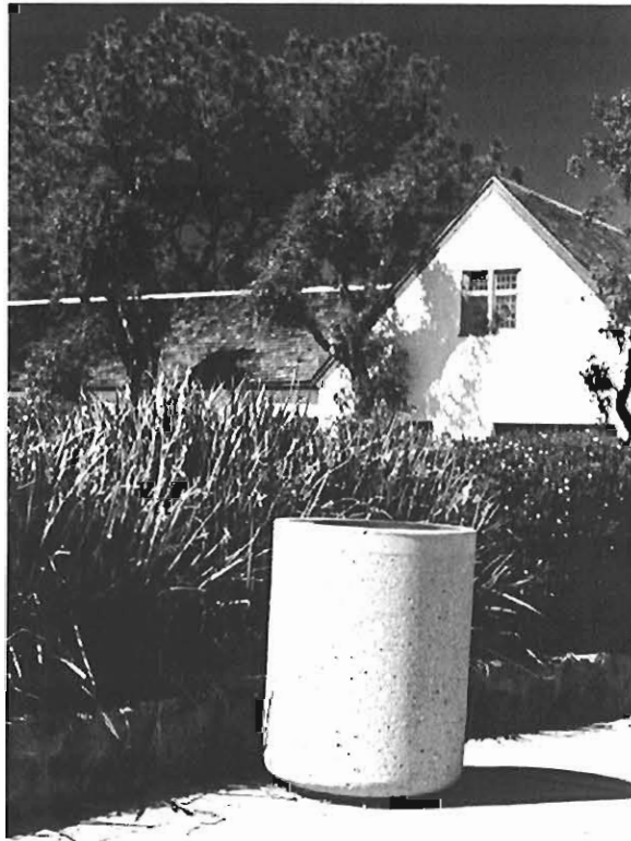
Existing trash receptacle of warm grey, colored concrete with light sandblasted finish and simple metal cover
