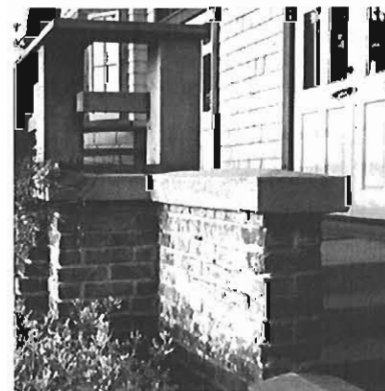
Brick wall detail with concrete cap and wood guard rails
