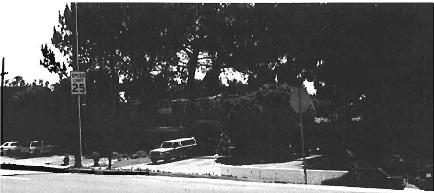
Motel site between 10th and 9th potential redevelopment with visitor-serving commercial and residential
