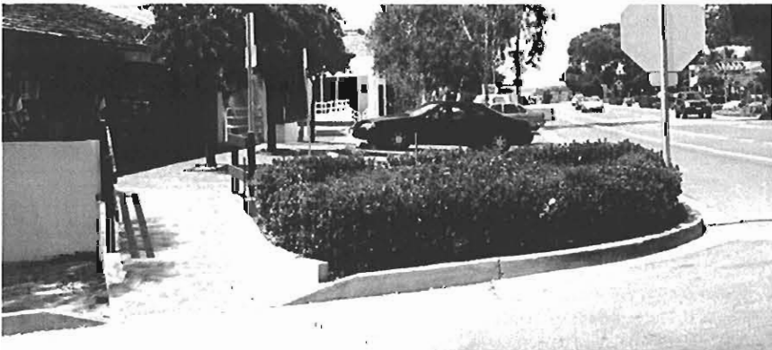
Ramp access at 11th Street is too steep
