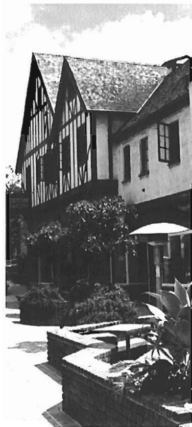
Corner of 15th Street and Camino del Mar
