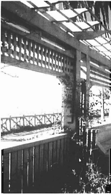
Trellis provides shade and creates a unique "Del Mar" style bus shelter
