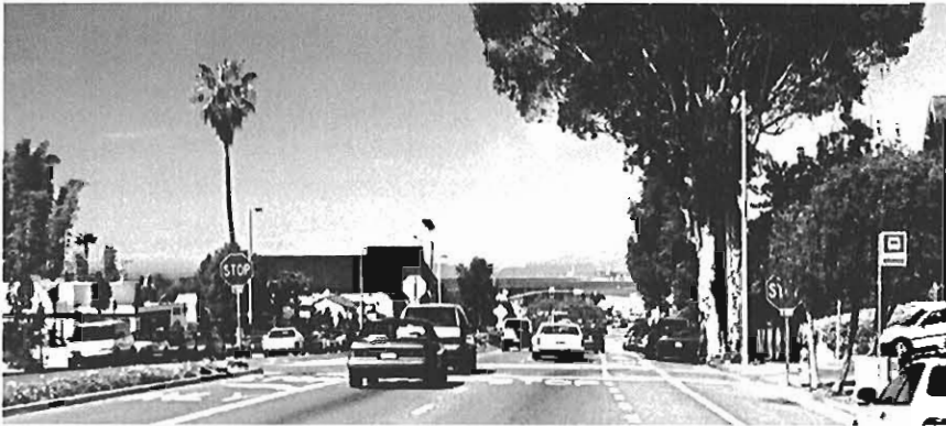
Excess lane width can be reduced for wider medians and larger pedestrian parkways
