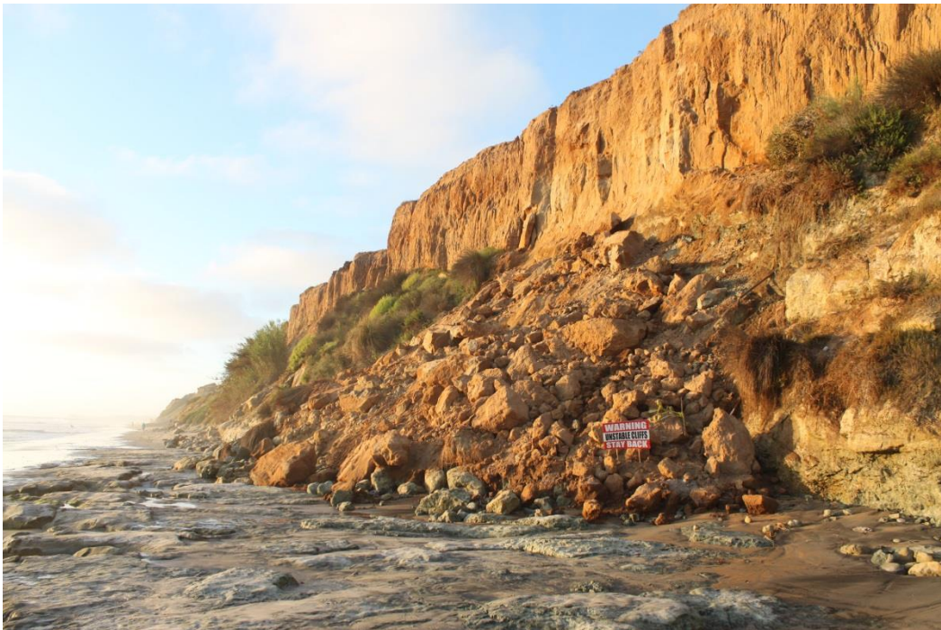
July 13, 2016 bluff collapse at 10 th Street
