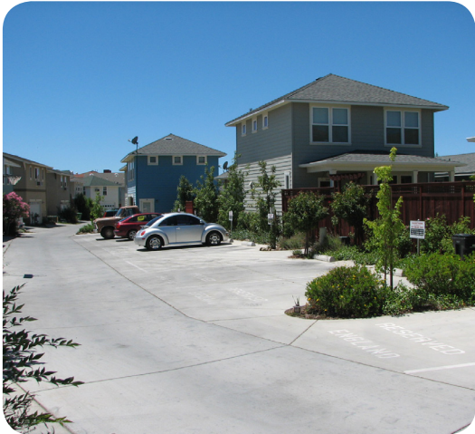
✗ Avoid large amounts of paving. Stormwater runoff should be directed to permeable areas.
