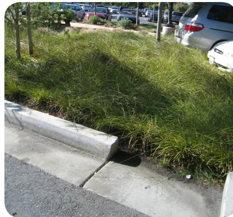
✓ Opening in curb allows for on-site stormwater to infiltrate in landscape areas.
