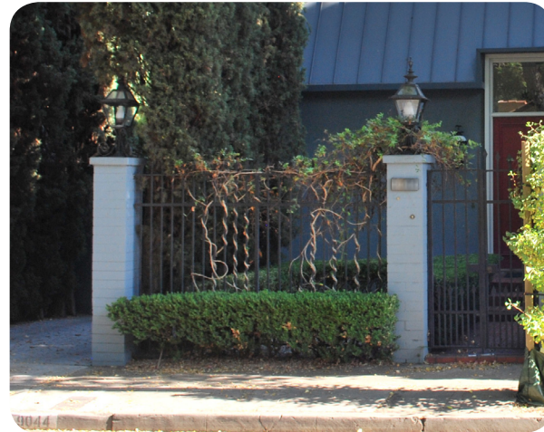
✗ Avoid unshielded style fixtures where bulbs are visible from adjacent properties or the public right-of-way.
