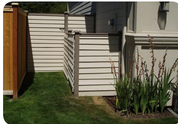
✓ Trash containers, mechanical, and electrical equipment should be screened from public view.
