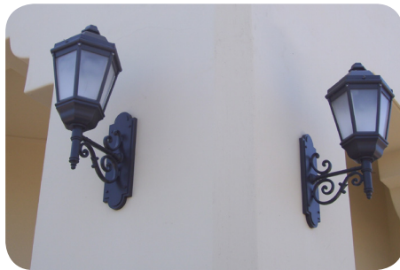
✓ Light bulb should be concealed and fully shielded. Utilize frosted or tempered glass.
