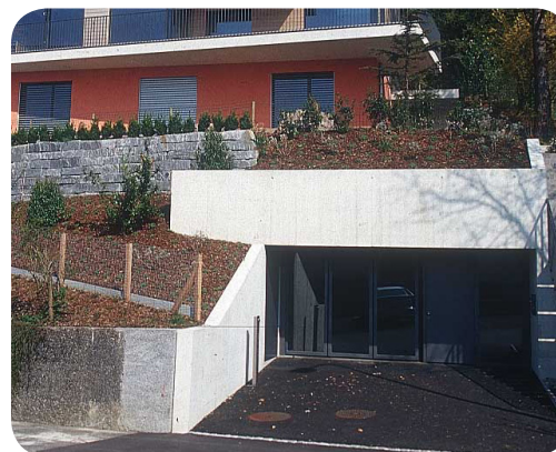
✗ Avoid massive land alterations that require large retaining walls.
