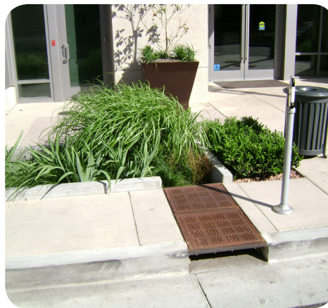
✓ Landscape strips are incorporated into the sidewalk to infiltrate stormwater runoff from the street.
