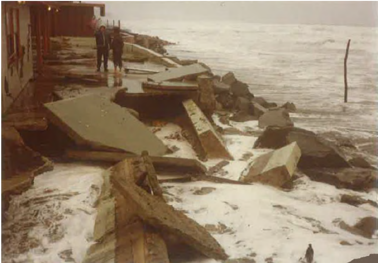
Figure 9.2 Coastal Damage Following 1983 Storm
