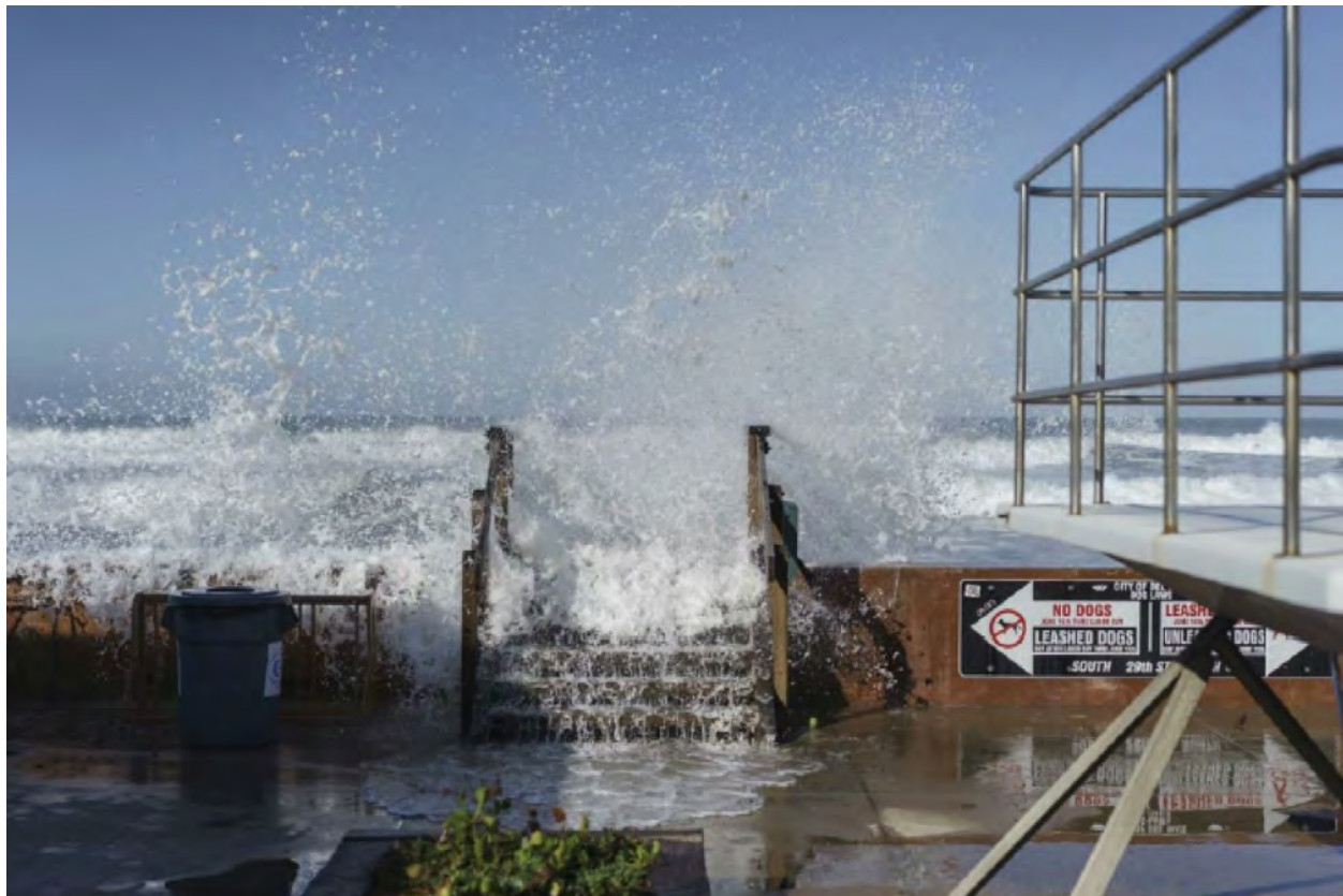
Figure 9.1 Overtopping in Del Mar on March 8, 2016
