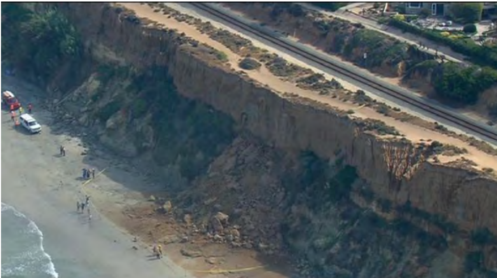
Figure 8.1 Bluff Collapse near 10 th St. in Del Mar on July 13, 2016
