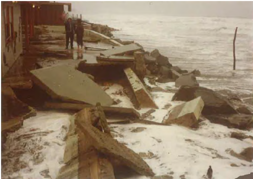
Figure 9.2 Coastal Damage Following 1983 Storm
