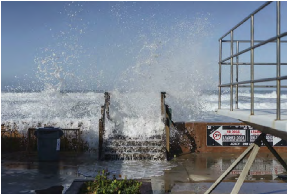
Figure 9.1 Overtopping in Del Mar on March 8, 2016
