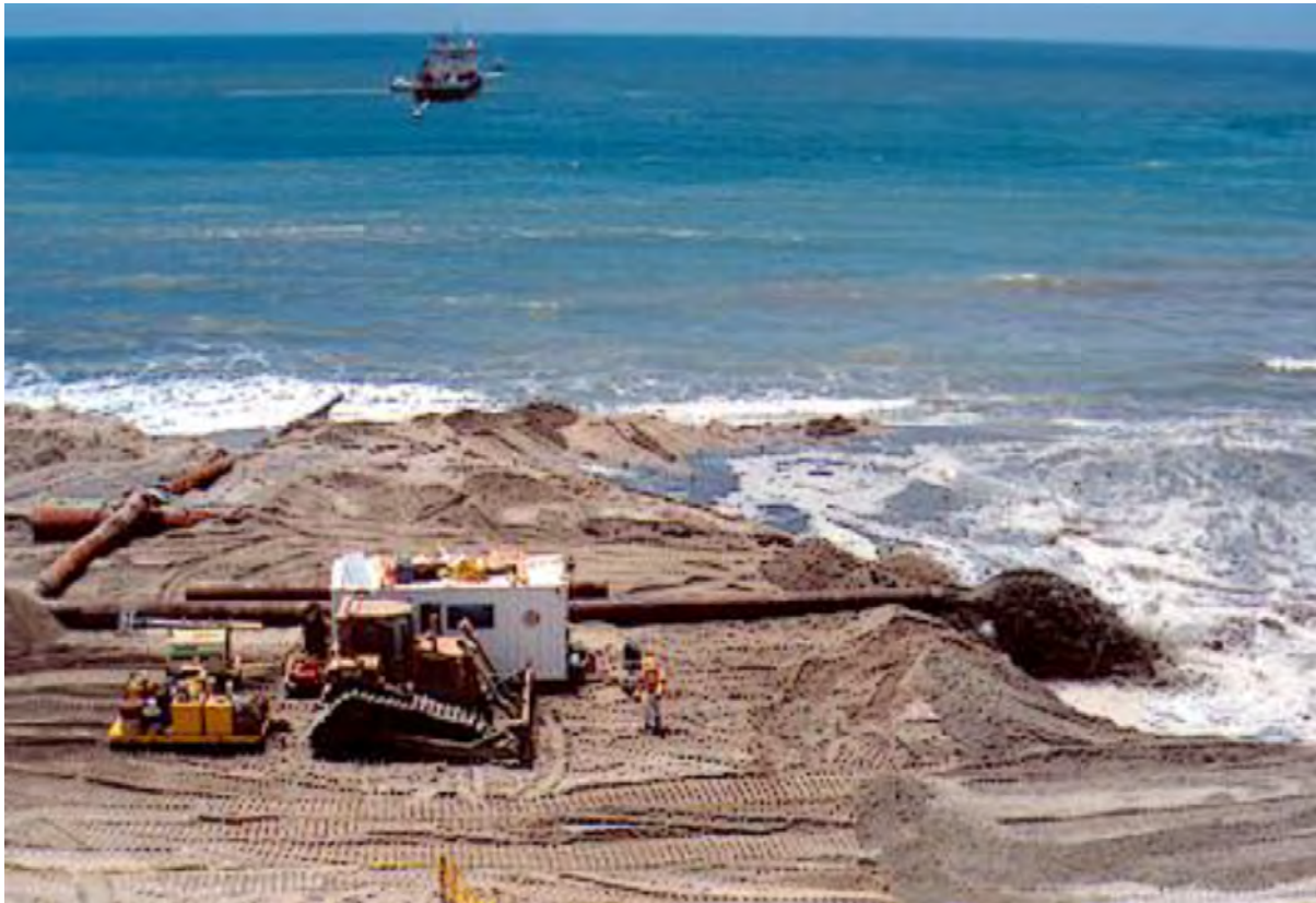
Figure 3.4.1.1 Beach Sediment Placement at Carlsbad
