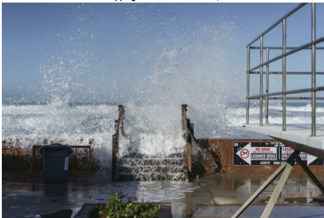
Figure 9.1 Overtopping in Del Mar on March 8, 2016
