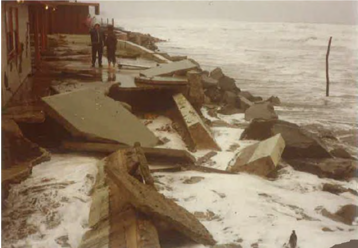
Figure 9.2 Coastal Damage Following 1983 Storm
