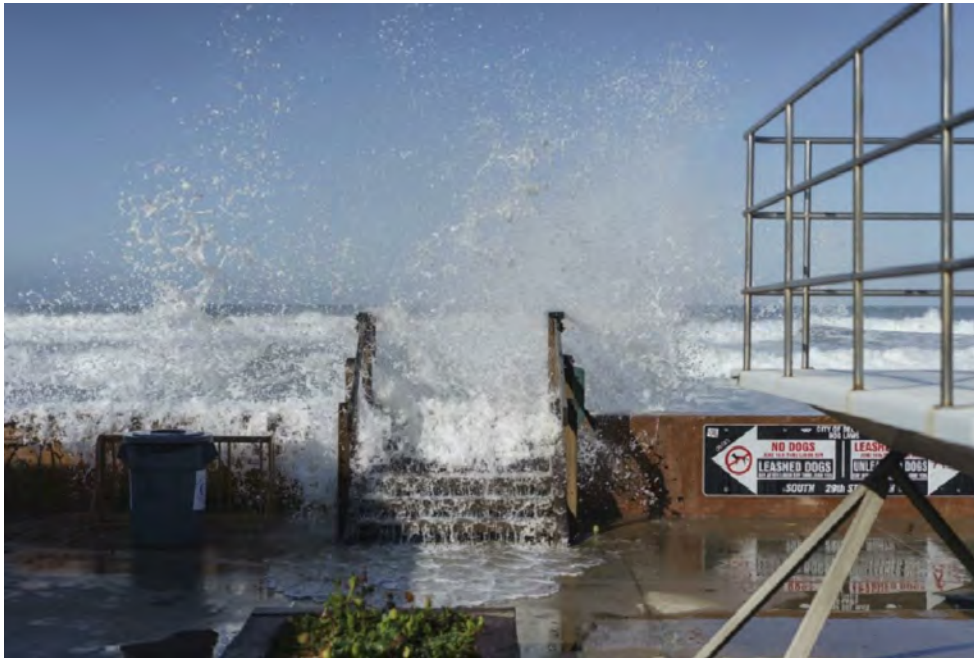
Figure 9.1 Overtopping in Del Mar on March 8, 2016
