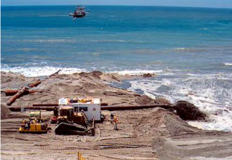
Figure 3.4.1.1 Beach Sediment Placement at Carlsbad
