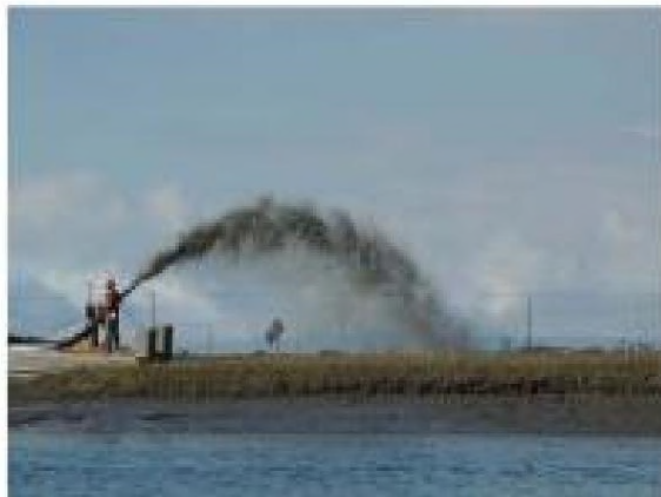
Figure 5.1 Sediment Placement on the Marsh at Seal Beach
