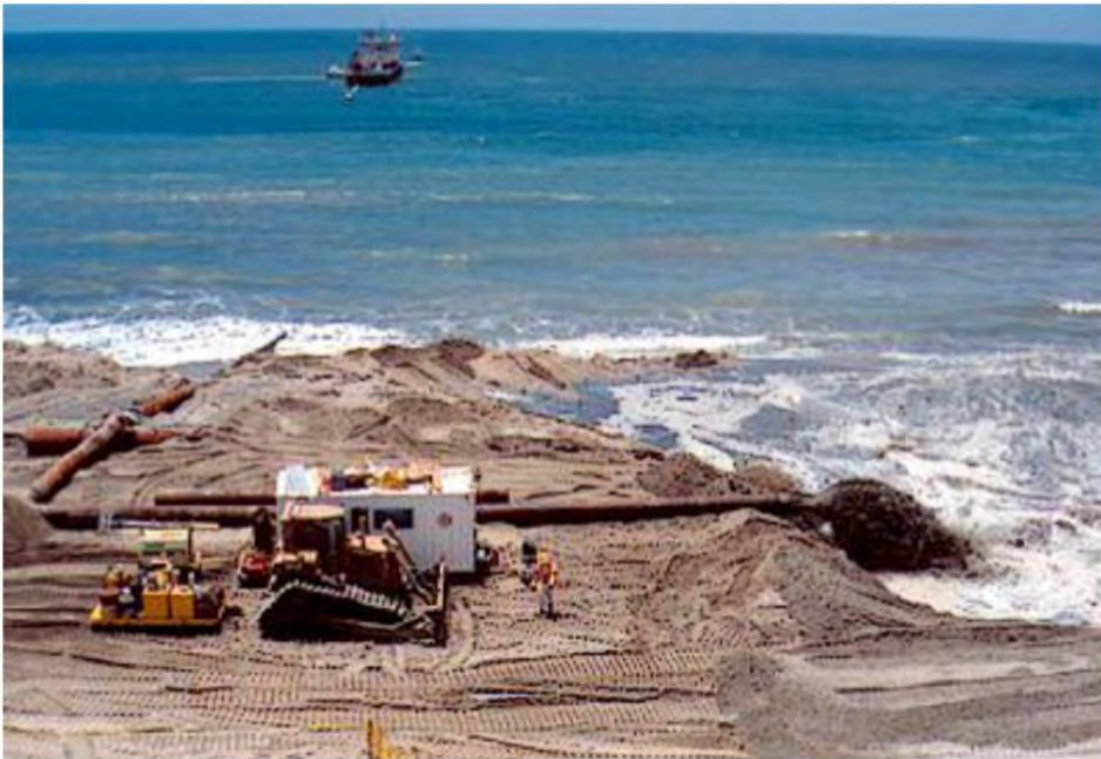
Figure B.4 Beach Nourishment, Dune Restoration, and Cobble Placement Illustration
