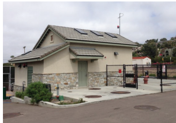
21st Street Sewer Pump Station
