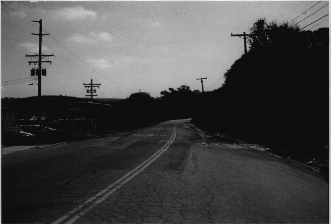
Photo location: Eastbound at start of segment
