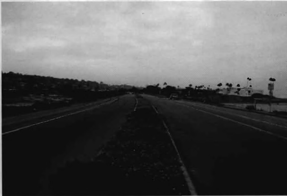
Photo location: Southbound at north of Bridge
