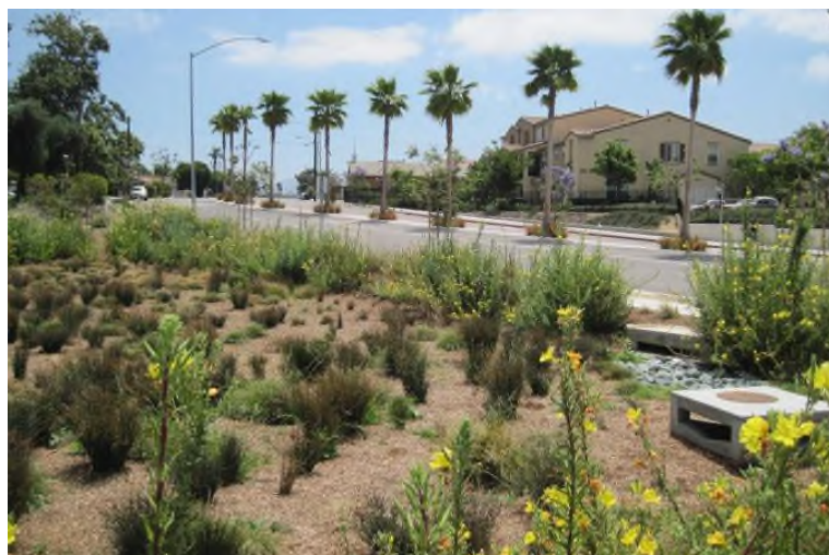
Location: 43 rd Street and Logan Avenue, San Diego, California
