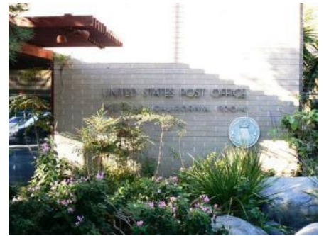
Del Mar Post Office, 122 15th Street
