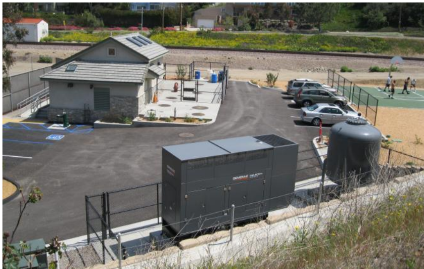
Del Mar 21 st Pump Station
