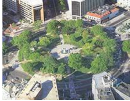
Older traffic circle
