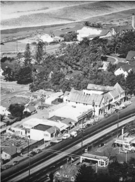
Del Mar's Village took shape in the 1930's and 1940's, which established the precedence for the proposed design regulations.
