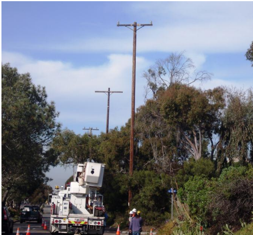
Utility poles were recently removed along Camino del Mar
