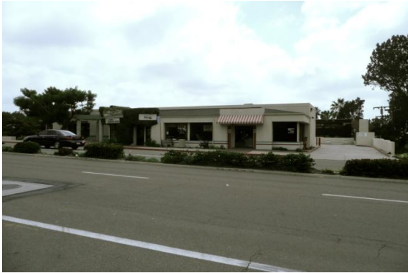
900 Block of Camino del Mar
