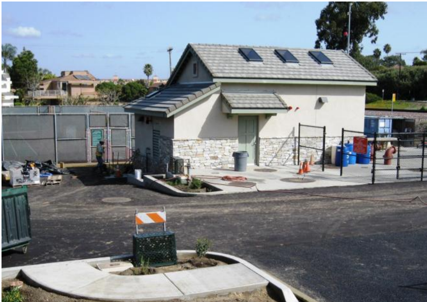
Del Mar 21 st Pump Station (under construction)
