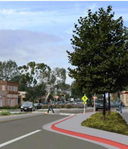
Roundabouts replace stop signs to keep traffic moving.
