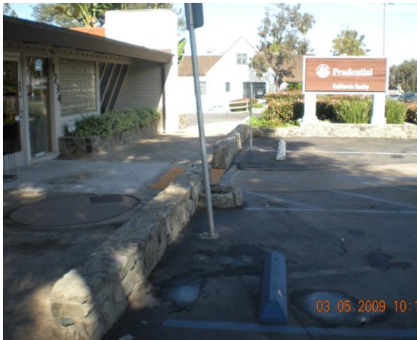
Town & Country stalls interrupt sidewalks
