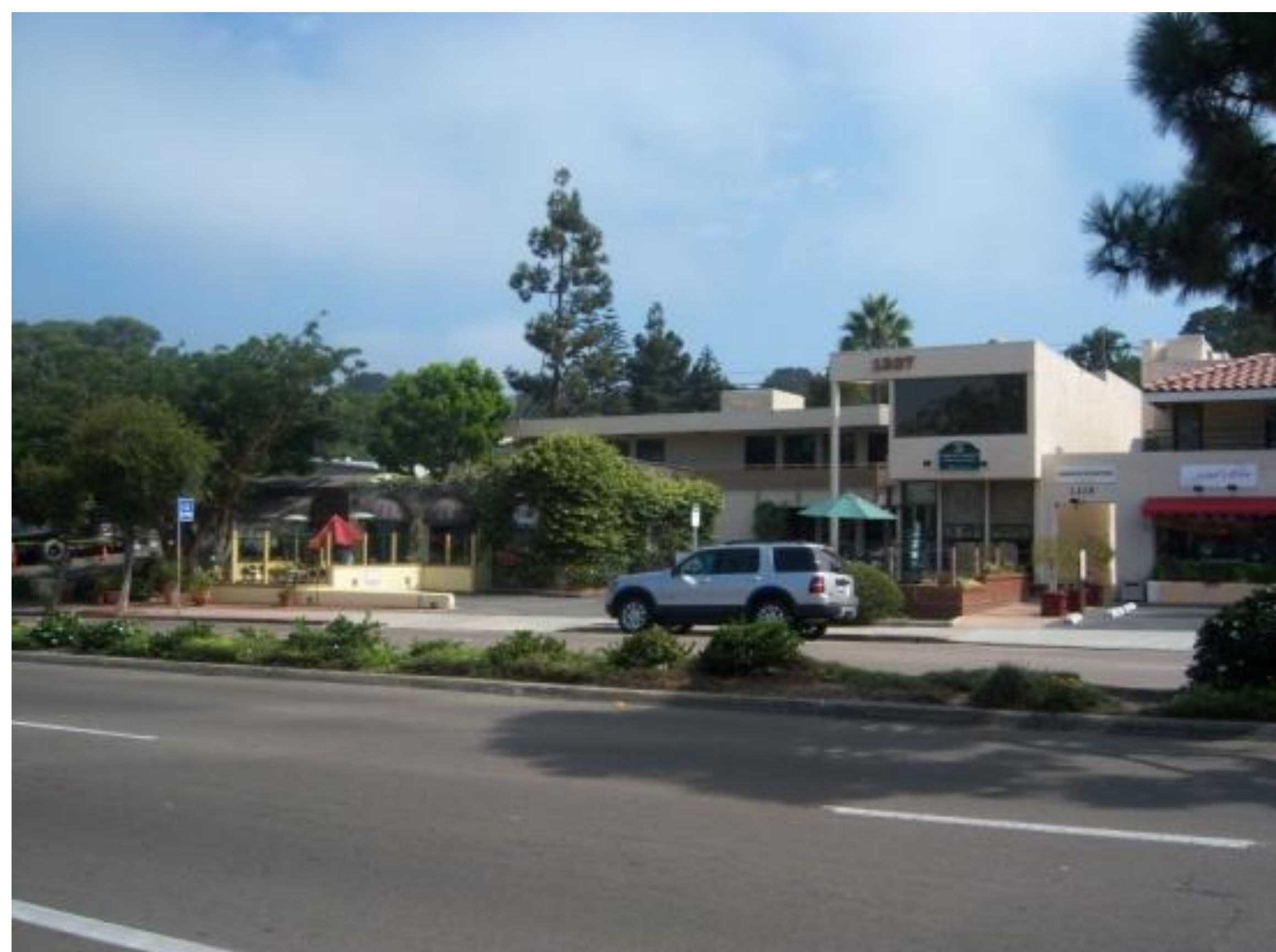
Oversized travel lanes
