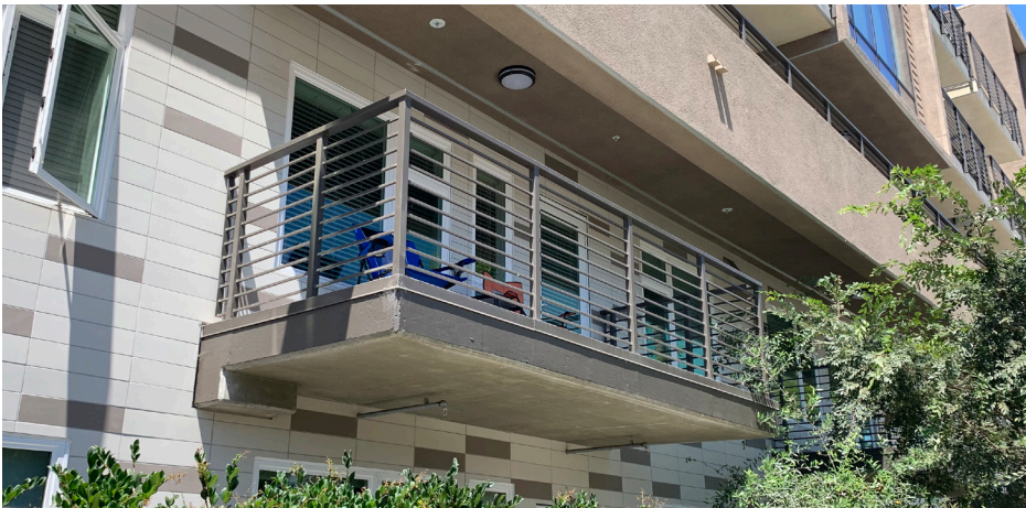
Private open space shall be no less than 5 feet in any direction.
