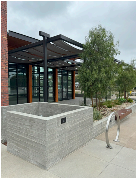
Screening of utilities with solid walls.
