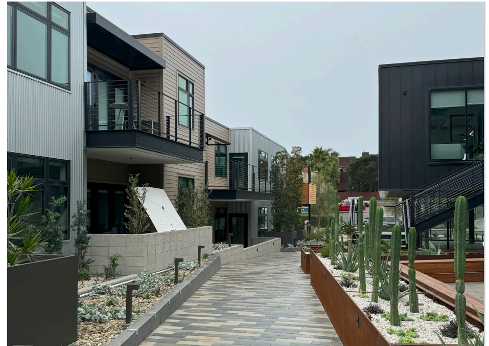
Common open space open to the sky, visible and accessible from residential units.
