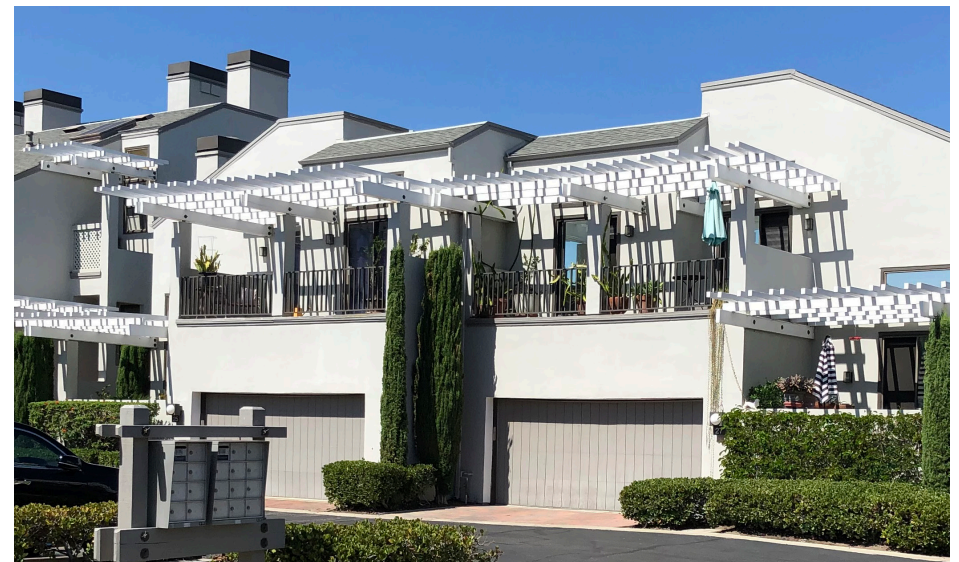
Recess garage doors to add shadow.
