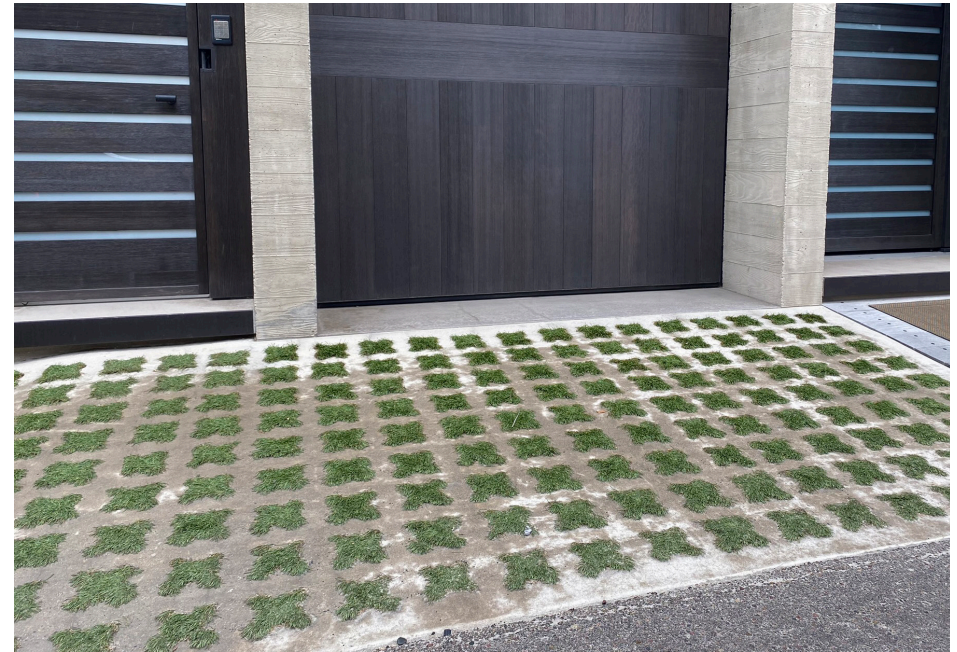
Permeable paving at a parking garage entrance.
