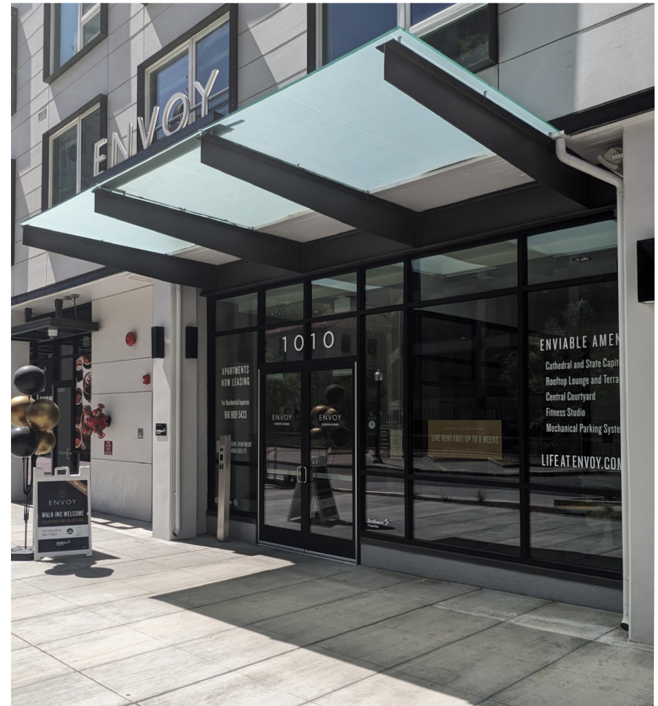
A shared entrance for all units of a housing development.
