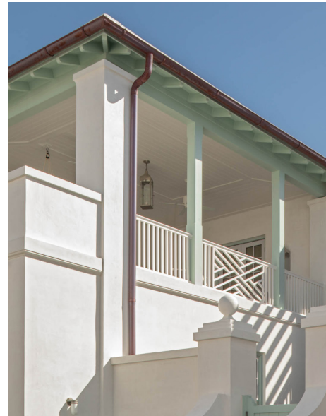
Decorative gutters matching roof.
