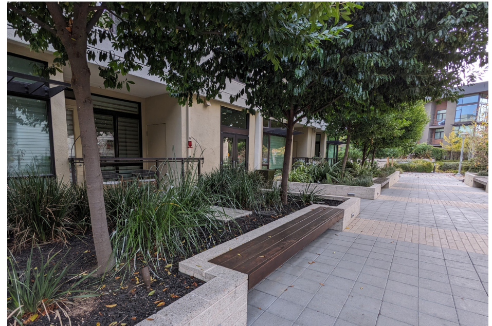
Public walkway paved with permeable pavers.
