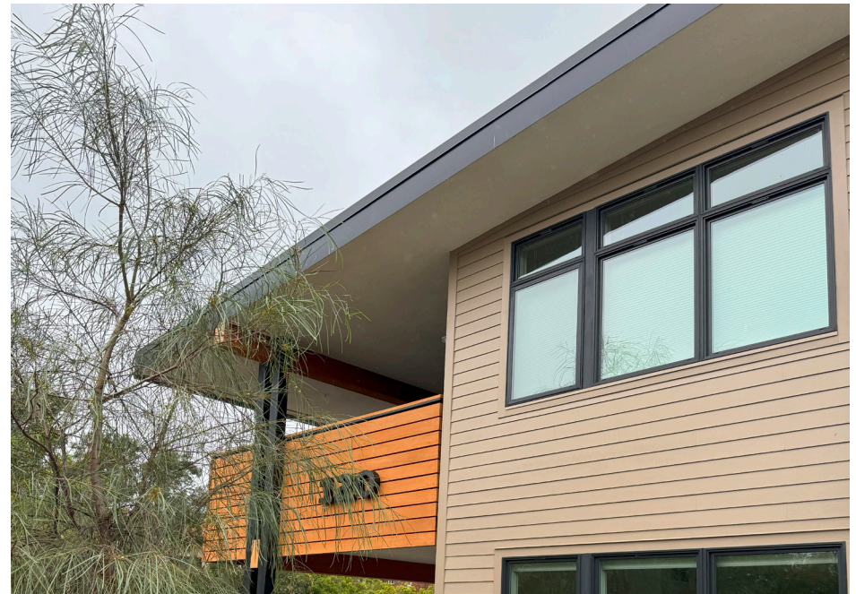
An example of a roof overhang.
