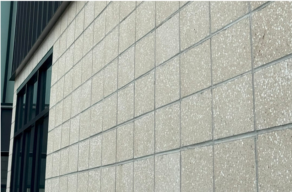
Concrete block used as an exterior finish material shall not be permitted.
