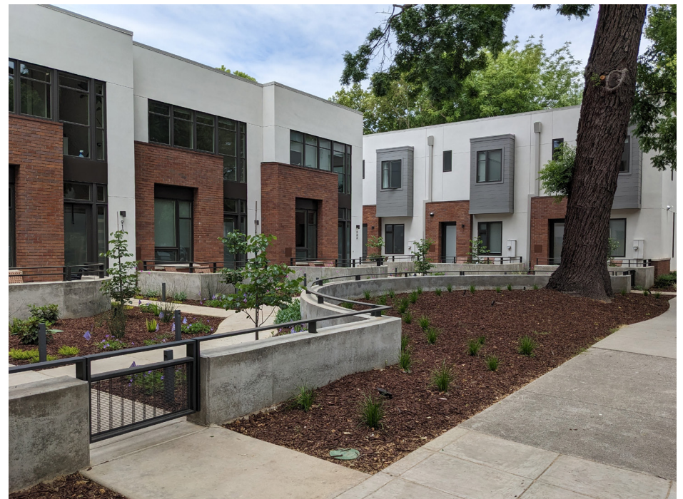
Seat walls between residential units and the sidewalk shall be 3 feet tall or less.
