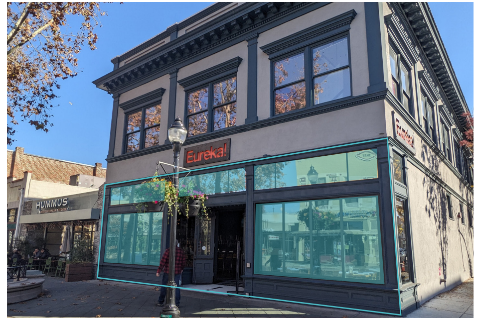
Commercial ground-floor facing Camino Del Mar shall be a minimum of 60% transparent.
