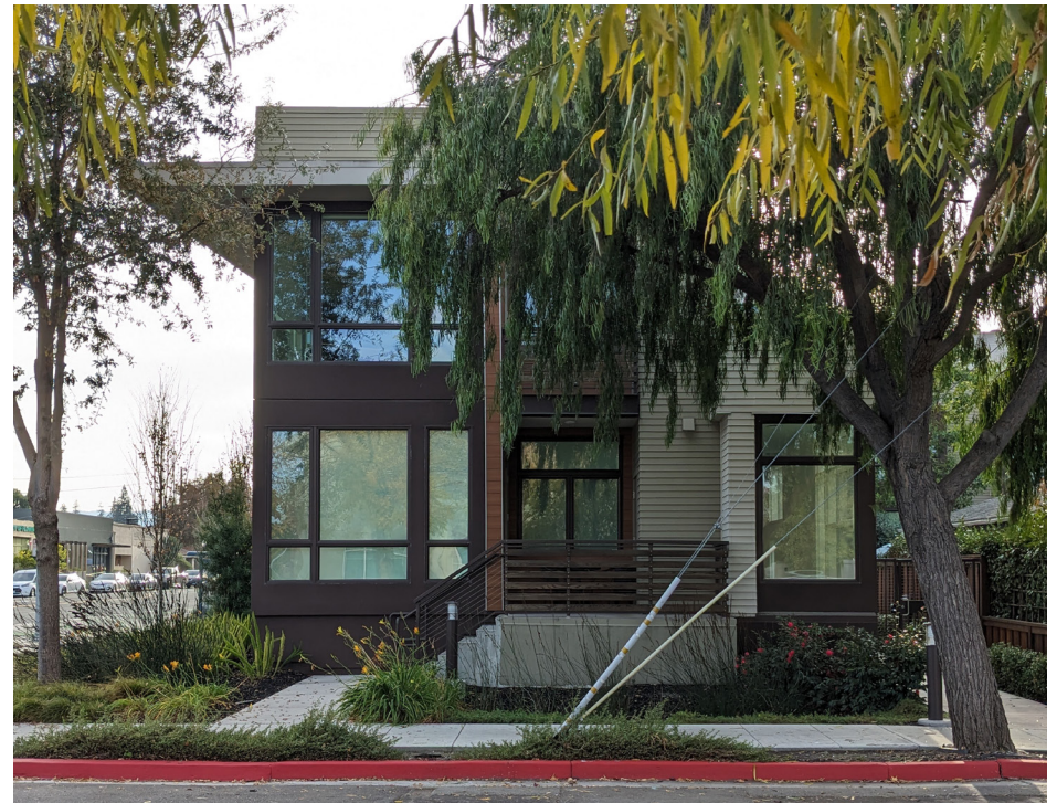
An elevated ground-floor with a stoop, planting, and matching material cladding along the foundation area.
